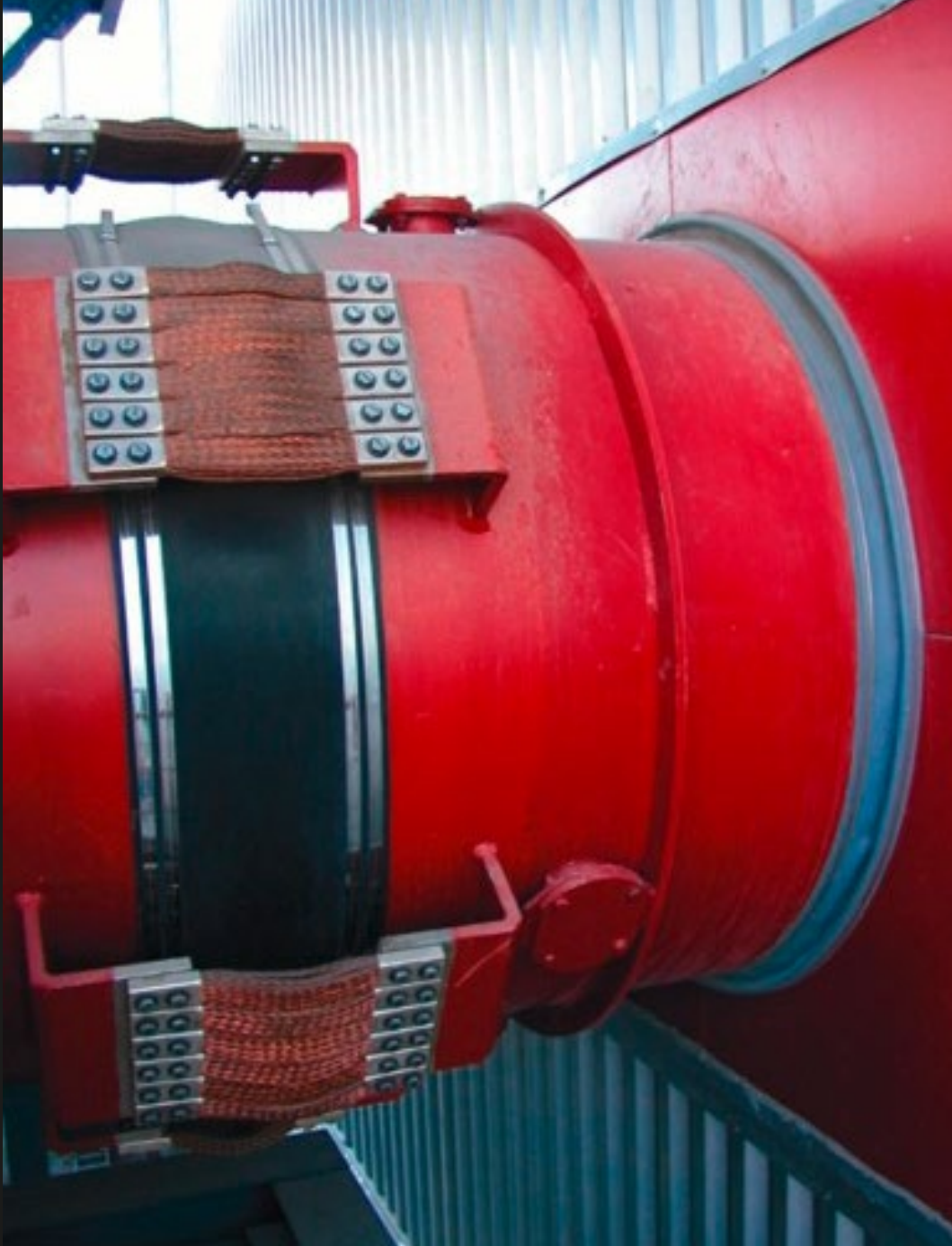
Pipe penetration seal and clamped EPDM rubber expansion joint penetration seal made from silicone rubber with open seam for afterwards closing on site
