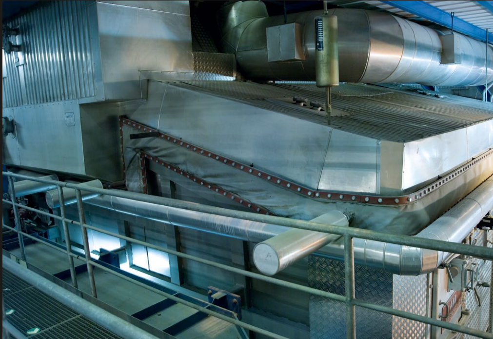
Multilayer expansion joint bellows, type GB300 as a seal between the grate and boiler in a waste incineration plant
