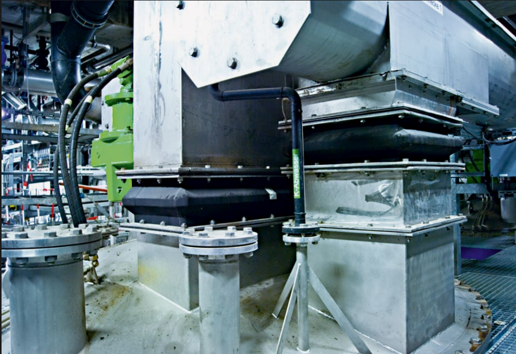
Elastomer expansion joints, type GU110 in the chute between the screw conveyor and sludge container in a slurry incineration facility ∅ 400 x 400 mm, 60 °C
