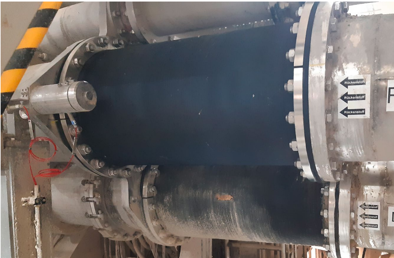
Replaced rubber flanged pipe in operation of a paper mill
