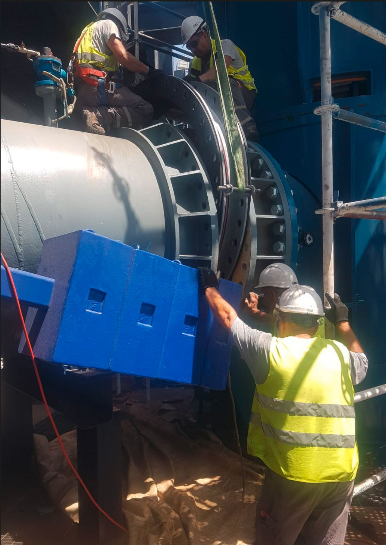
Installation of a rubber expansion joint Ø 1,600 mm to the pump nozzle, 16 bar design pressure
