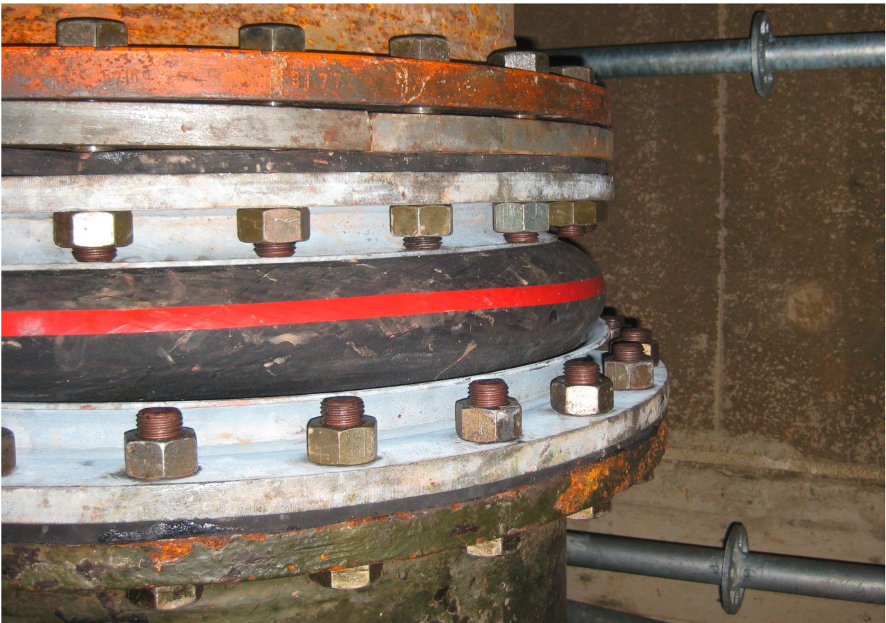
Rubber expansion joints with built in lateral offset to compensate pipeline misalignment
