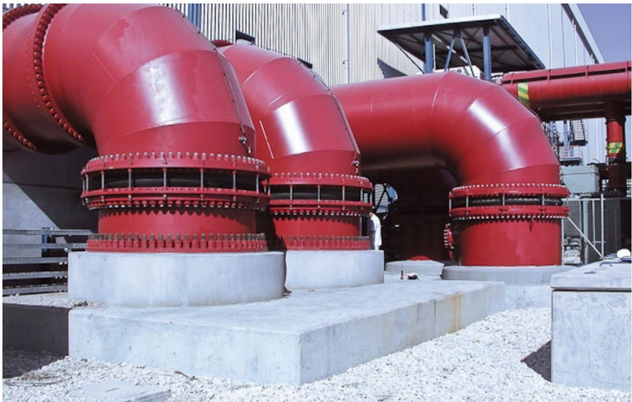
Sea water intake cooling water line Ø 2,600 mm, operating pressure 2.5 bar, lateral tied rubber expansion joints of type U111M
