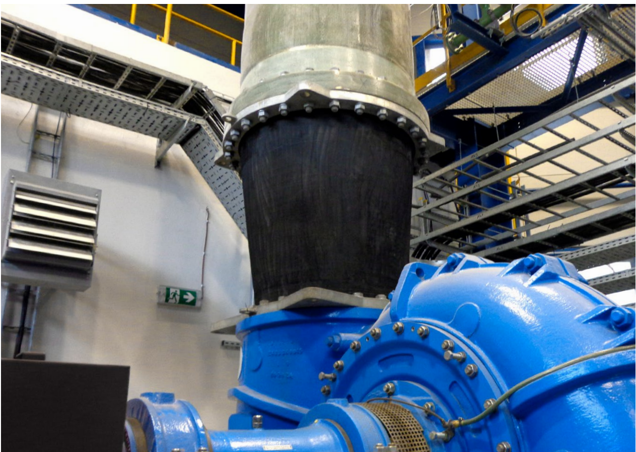
Conical expansion joints, type U300A on the suction and discharge side of a gypsum slurry pump in a desulphurization unit of a power plant
