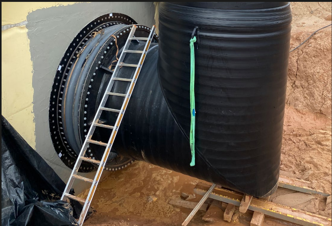
Ø 2,600 mm double arch ground water penetration seal made from radiation resistant silicone rubber installed outside of a building design pressure 20 m WC, lateral displacement 60 mm from building settlement
